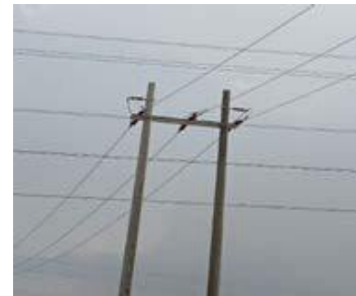
55km 33kv double circuit distribution lines project
