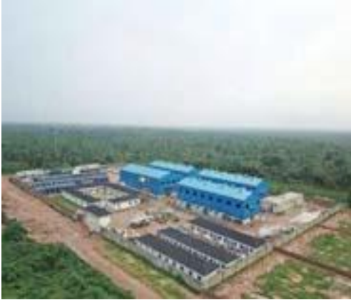
Osiommo - 55MW Generation Project
